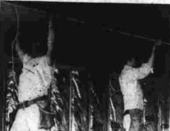
radiant heating ceiling. Installed like a regular gypsum drywali ceiling, it's available in 6, 8, 10 and 12 foot lengths. Each Panelectric panel has its own particular combination of heat
